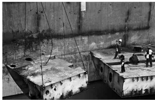
(Left) The final stages of recycling, double bottom sections are removed while the next ship is alongside, and (right) after 12 weeks small steel strips are all that is left.
